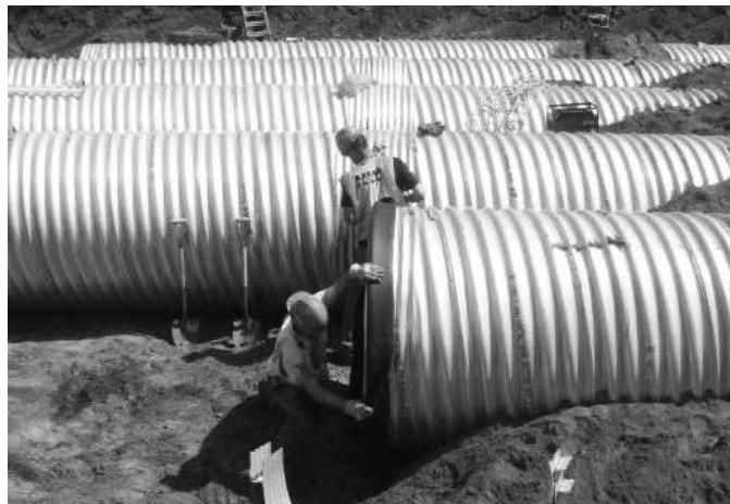
*Installation of band with flat neoprene gasket.*
