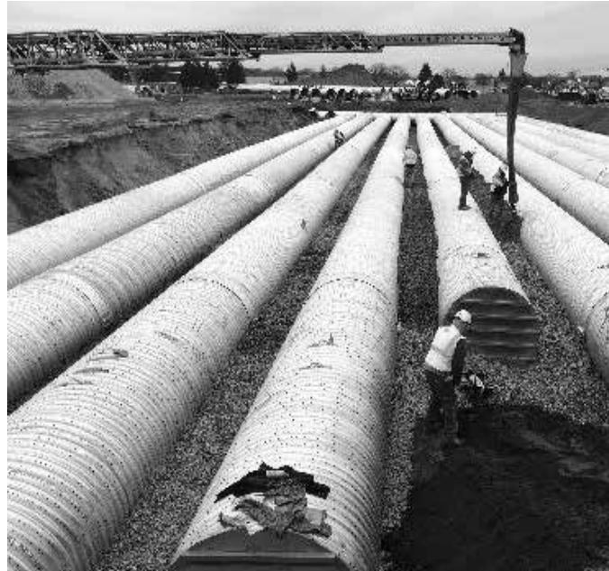
Placing backfill with a conveyor.
