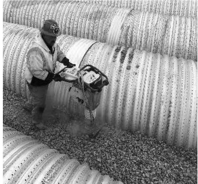
Compaction with vibratory equipment.
