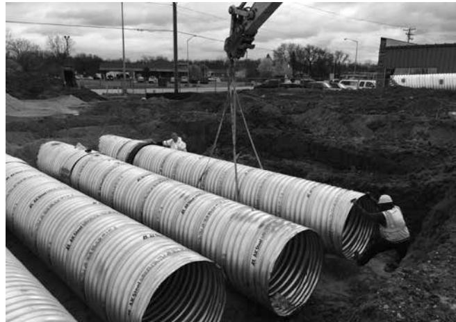
*Lifting ALT2 CMP with nylon slings.*
