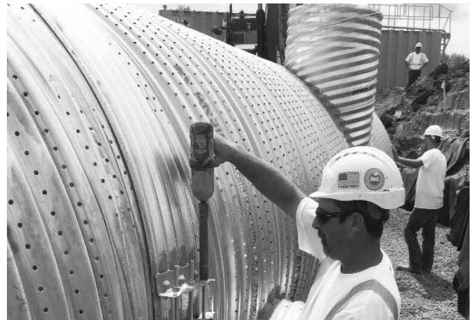
*Tightening bolts on a corrugated band.*
